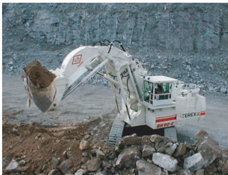
Figure 17.3. O&K RH90C Excavator
