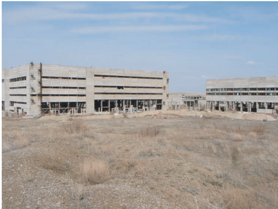
Figure 4.2. Existing processing facility at the Chilisai project site
