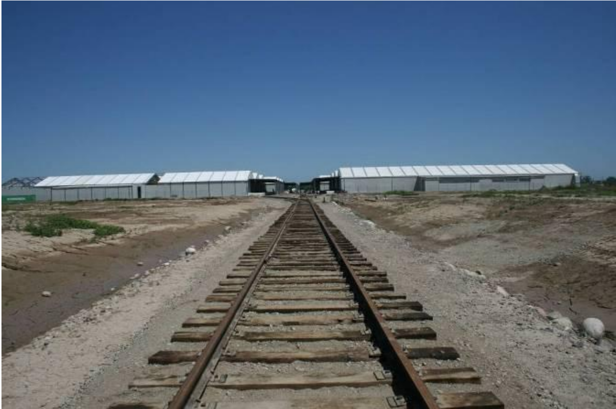
Railway leading to the warehouses
