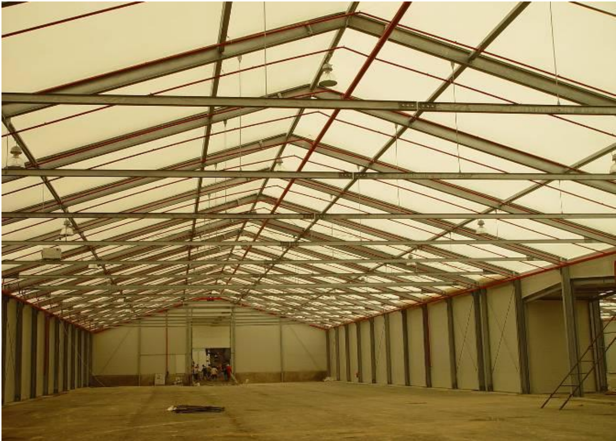
Interior of warehouses under construction
