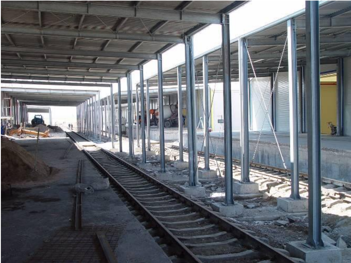
Warehouses under construction
